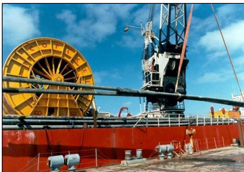
Figure 9: Pipeline Cut into Sections for Recovery
